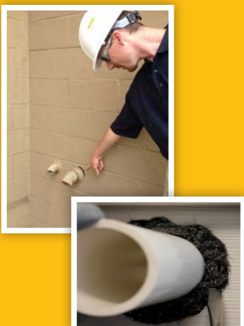
Exterior Inspection and Pest Proofing
